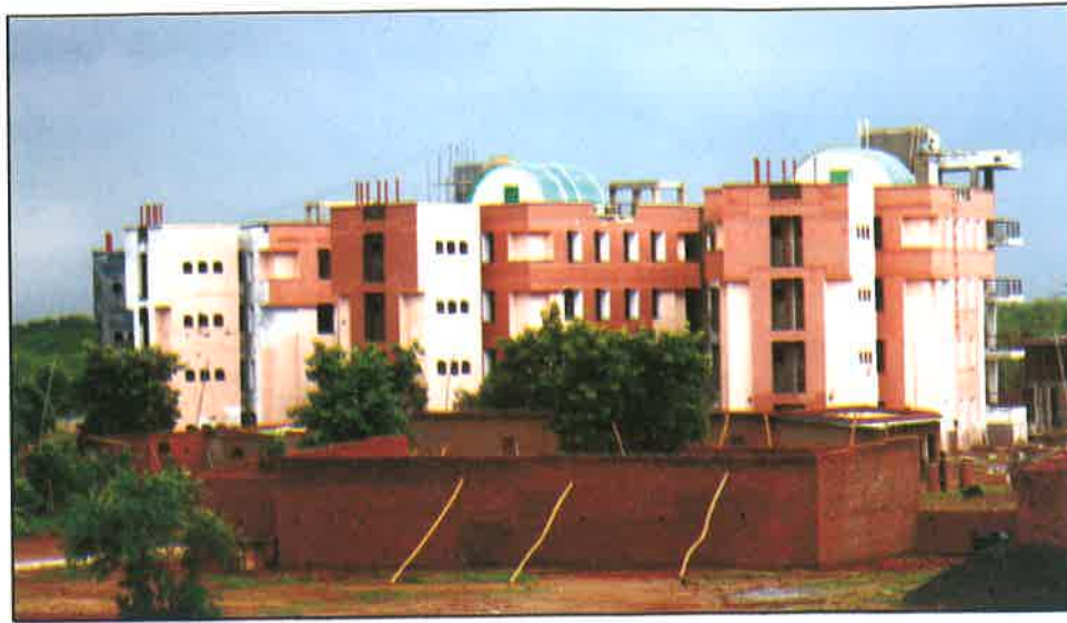
Triple Seated Hall of Residence 1 (Under Construction)
