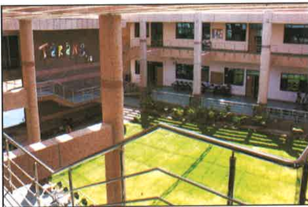
Core Lab Complex, Inside
